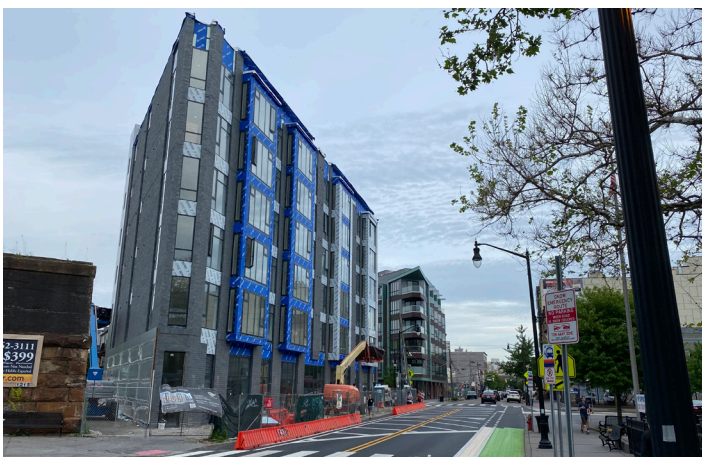
New 5 over 1 buildings under construction. Courtesy Dennis Pierce
