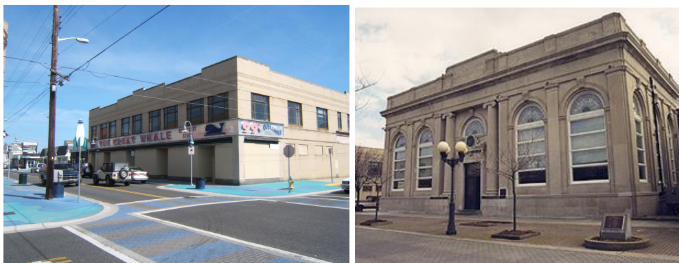
Figure 6. The G.C. Murphy Building (The Great Whale 99 cent store) MLH Figure 7. Crest Savings Bank (Wildwood Historical Society, Inc.)
